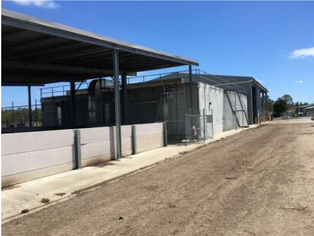
FIGURE 2-2 BIOFILTER, TUNNEL COMPOSTERS AND SHREDDING BUILDINGS
