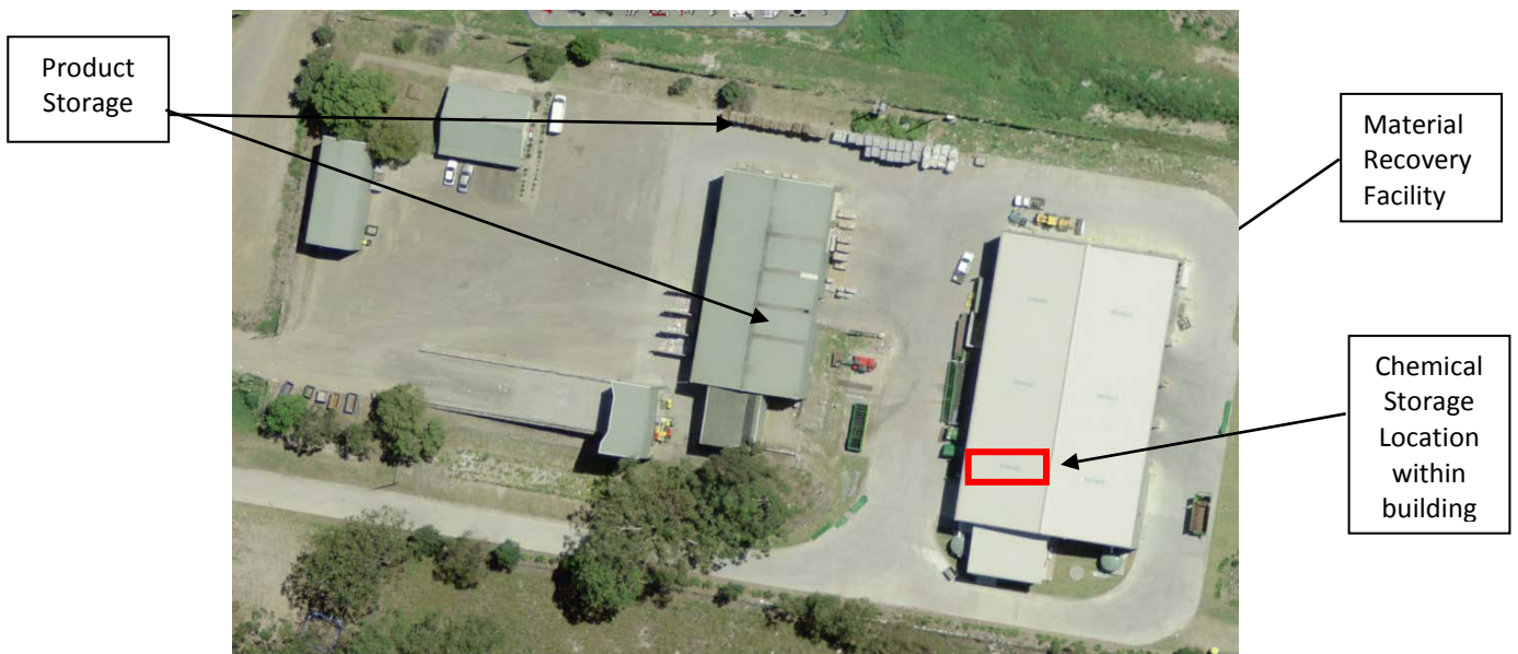
JR Richards Material Recovery Facility
