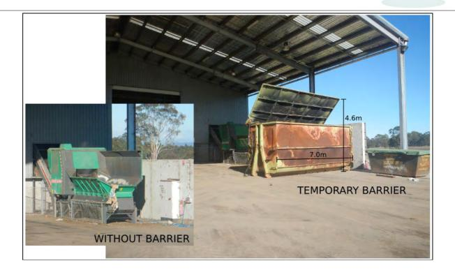
Figure 5.1 - Temporary Barrier
